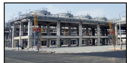
Shell & Fin Tube Heat Exchanger
